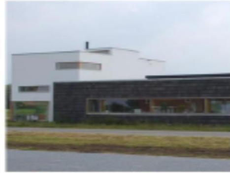
Roof tile as the outside wall of a temporary sales office
