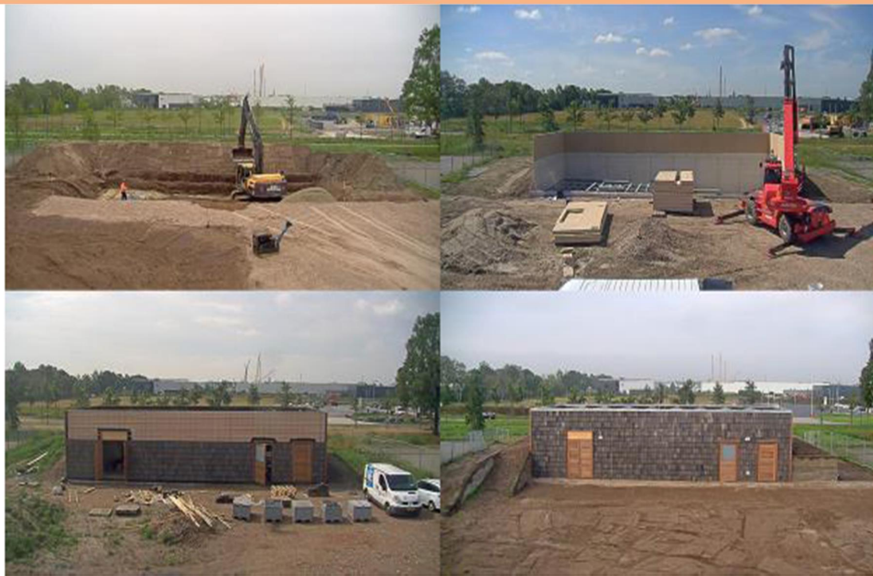
Figure 3: re-use of excavated soil, wood frame construction, prefabrication.
