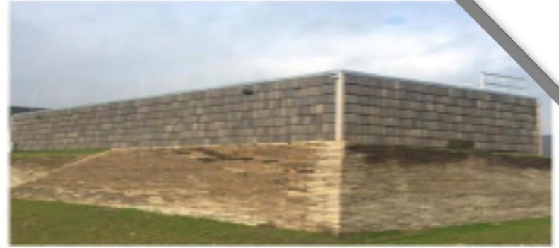
Roof tile as outer wall of substation
