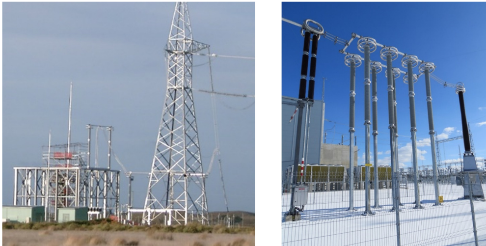
Figure 2: Outdoor DC transition yard OHL to cable(left), Paralleling of arresters for DC cable protection (right).
