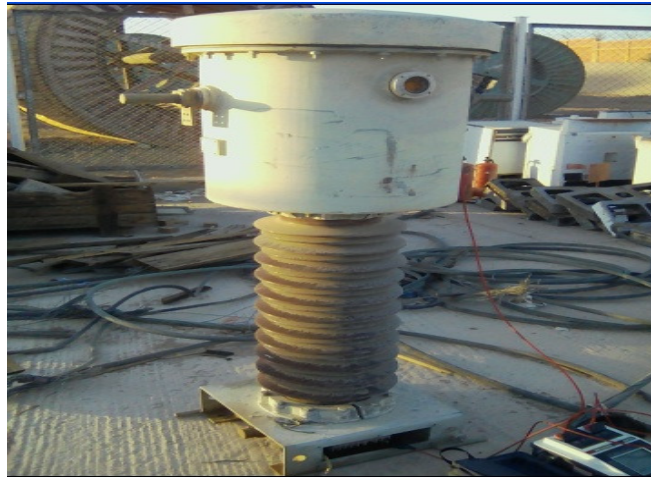
Figure 1: The current transformer was used.
