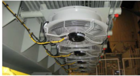
Figure 8: First 40/50 MVA, ONAN/ONAF grid coupling transformer with new speed-controllable fans with EC technology manufactured in Germany in 2009
