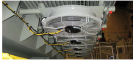
Figure 8: First 40/50 MVA, ONAN/ONAF grid coupling transformer with new speed-controllable fans with EC technology manufactured in Germany in 2009
