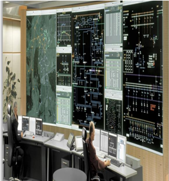
Remote HMI (NCC)
