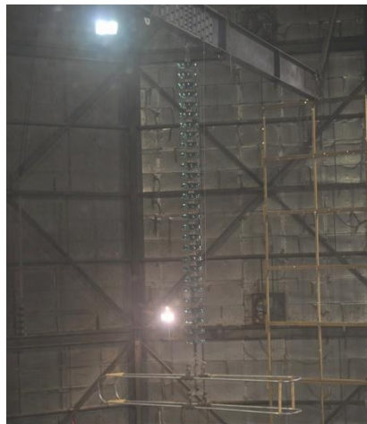
Figure 3: A replica of the Cahora Bassa pylon dimensions in the EPRI HV laboratory
