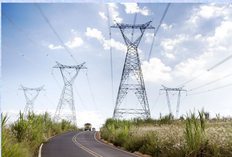
January 13, 2017 - Ultra-high-voltage transformers to help deliver clean hydropower via Belo Monte link to ten million people
