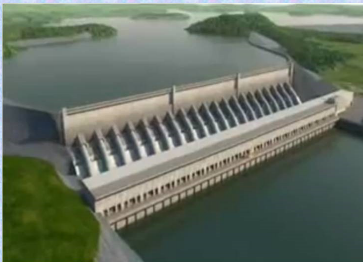
Belo Monte hydroelectric project
