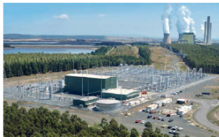
LCC Converter Station, Courtesy Siemens
