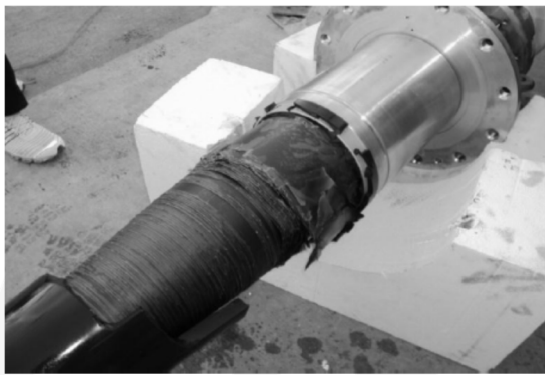
Oil-side porcelain part of GT21 main transformer (red phase) high voltage bushing after incident
