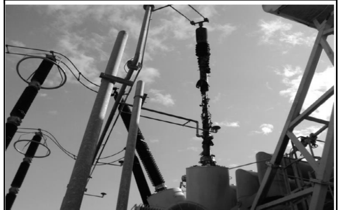
GT21 main transformer high voltage bushing (red-phase) explosion incident
